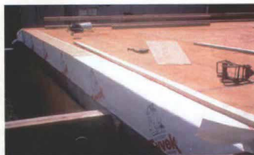
Wrapping the rim joist in Tyvek and then sealing the vapor barrier to it traps interior air but allows moisture to escape.
